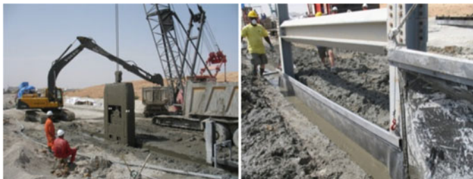
Fig. 1 Excavation of a trench
